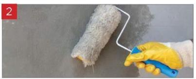
If we are installing on an absorbent substrate such as plasterboard or wood, we must apply **VIODOM BIO ACRYL B-13** primer to reduce absorbency.
