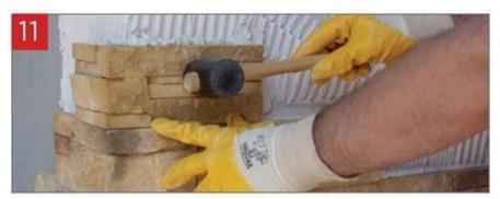
When installing the stone, use a rubber mallet to avoid damaging the stone.
