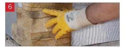
If the installation involves corners, start at the corner of the wall and continue the installation according to the flat elements.
