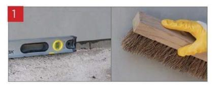
We clean the substrate from dust and dirt, for good adhesion of the mortar. Place the first line where the stones will be placed.
