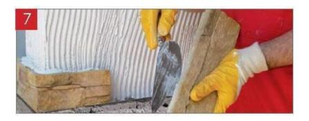
Using the trowel or rebonding tool, clean the perimeter of the stone from overlapping concrete for better installation. Since the back surface of the stone is dry, moisten it with water to prevent water absorption by the mortar.
