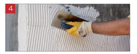
Apply MATHIOS STONE Extra-Stone-Glue 25kg mortar to the installation surface as needed to prevent it from drying out during stone installation.
