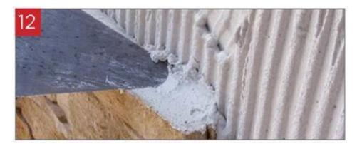
Fill the perimeter channel of the stone with glue using the trowel. Remove any excess glue using a towel.
