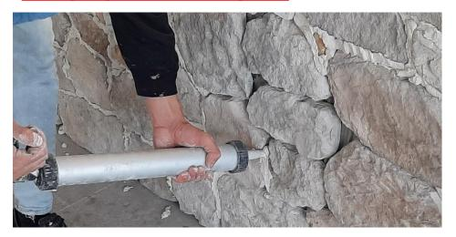
Stone grouting with <u>Mathios Grout by MATHIOS STONE</u>, offering the ability to fill grouts from 10mm to 50mm and is suitable for installation to interior and exterior surfaces. The application should be done with an <u>ORION X7-1000</u> gun suitable for coarse-grained grout.
