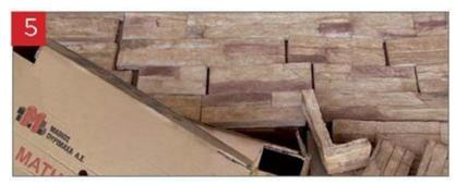
Place stones and mix from several cartons of at least 2m<sup>2</sup> to create a balance between different colors, shapes, thicknesses and textures.
