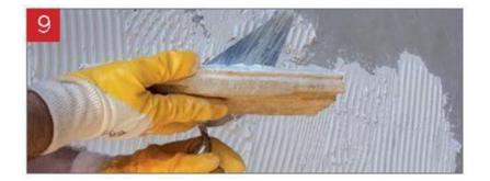
Apply the glue to the back surface of the stone as much as possible so that there is no gap between the stone and the surface.
