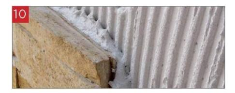
Place the stone by pressing hard to ensure a very good adhesion of the glue to the back surface of the stone.
